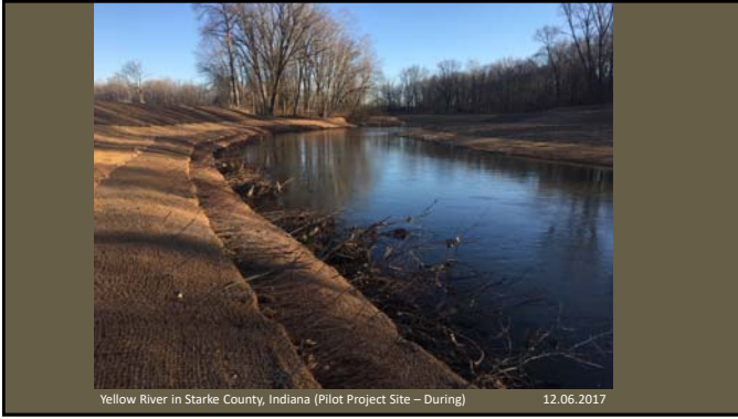
Yellow River in Starke County, Indiana (Pilot Project Site - During) 12.06.2017
