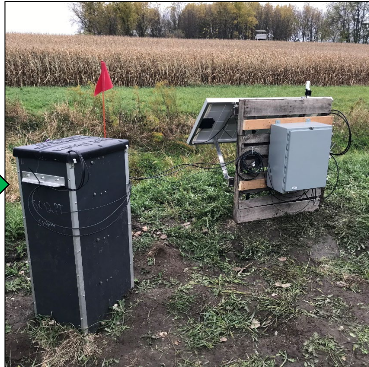
Continuous monitoring V-notch weir, pressure transducer, datalogger, ISCO
